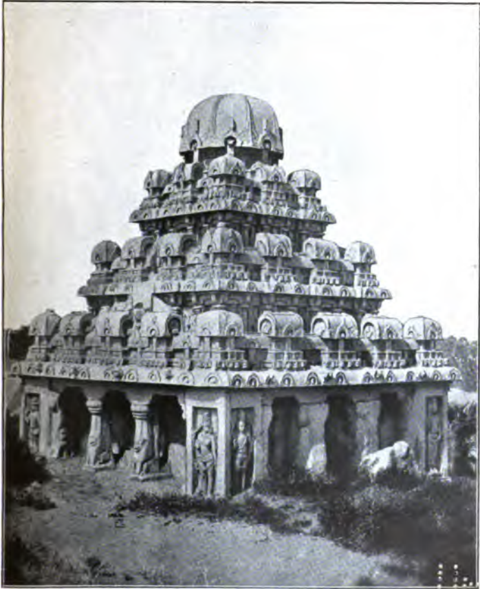
DHARMA-RĀJA RATHA AT MAMALLAPURAM
